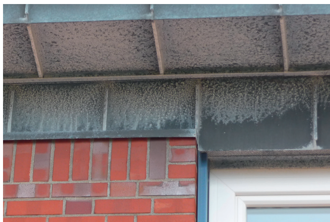
Examples of salt deposits on soffits and undersides of gutters
