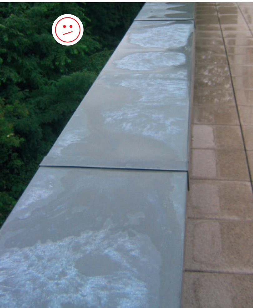
Zinc hydroxide formation due to insufficient slope
