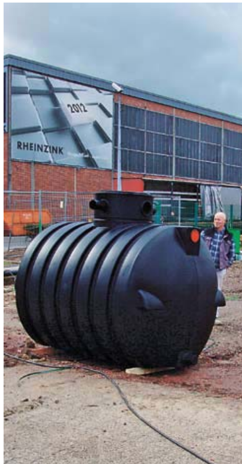
Installation of the nautilus rainwater tank (4 m 3 )
