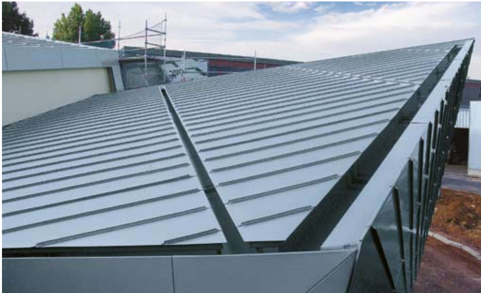
Roof structure with integrated roof drainage
