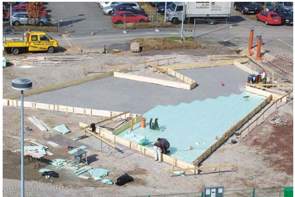
Work on the ground slab in progress
