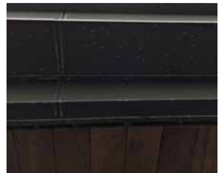
Examples of salt deposits on soffits and undersides of gutters
