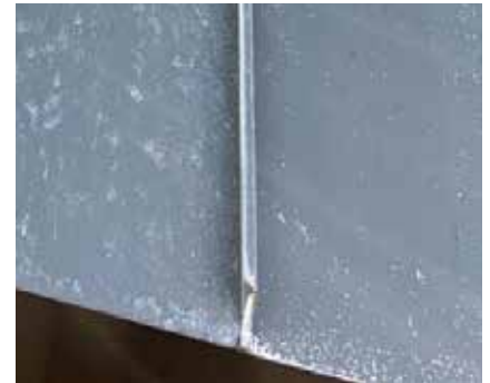
Examples of salt deposits on façades, seams and drip edges
