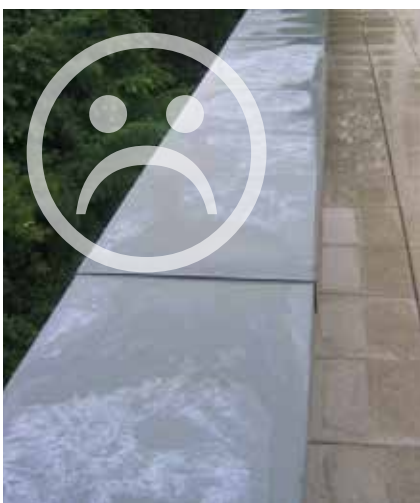
Zinc hydroxide formation due to insufficient slope
